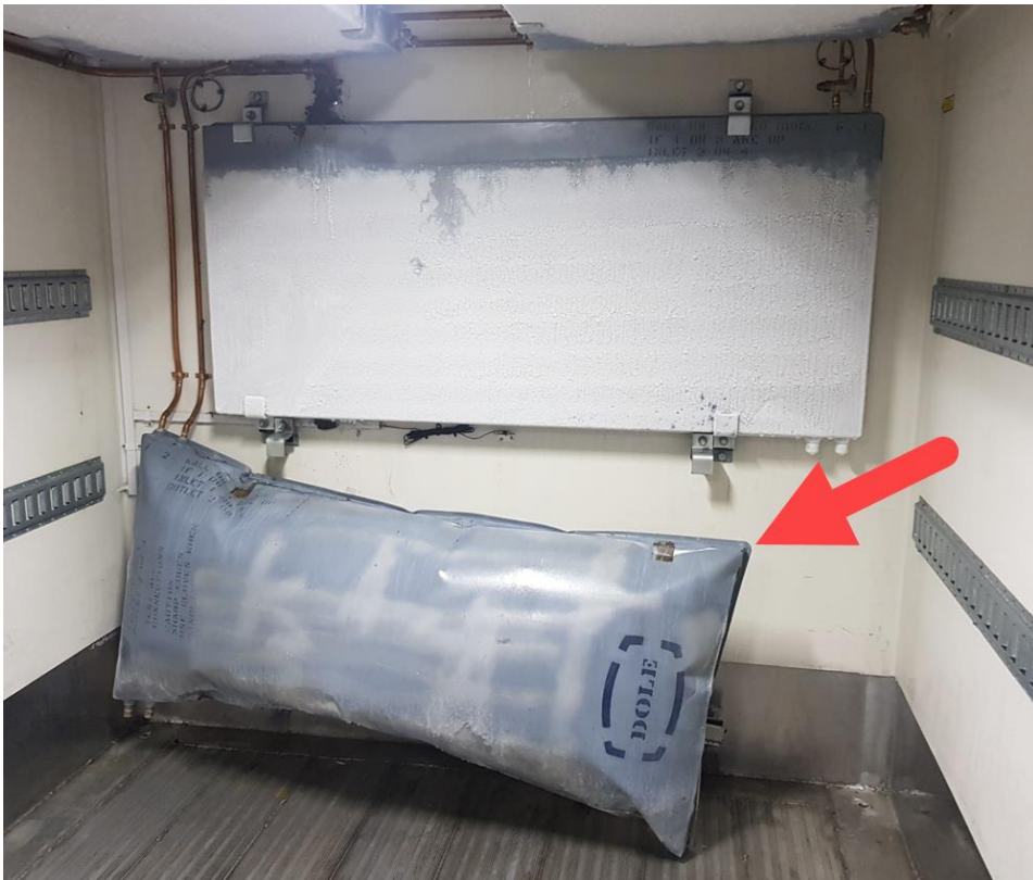
Figure 7: Cold Plate with internal refrigerant leak, fell out of plate brackets.
