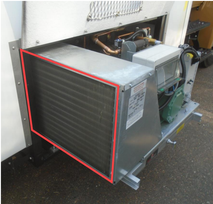
Figure 6: Condenser Coil location on a skirt-mounted condensing unit.
