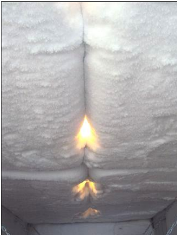
Figure 3: Example of extreme frost accumulation.
